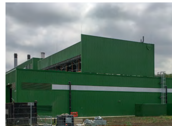
Holbrook Community Renewable Energy Centre air cooled condensers intake visible as linear slot on elevation
